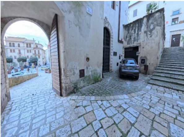
36 Internal entrance portal and ramp
