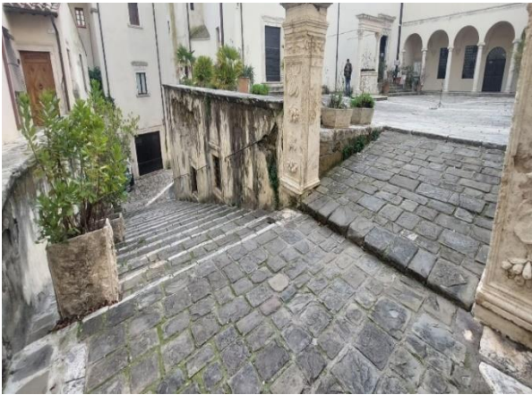
37 Staircases and final ramp
