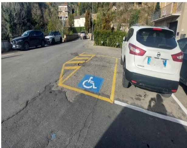
1 Reserved parking Via S. Chiara
