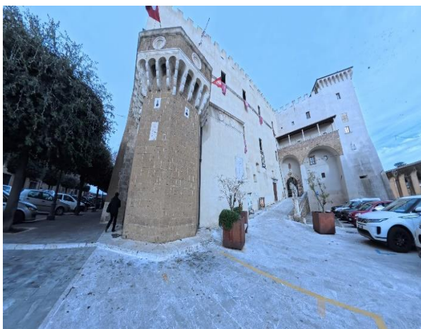
33 Entrance ramp to the Fortress Portal
