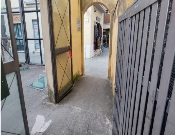
52 Access ramp Rubble area
