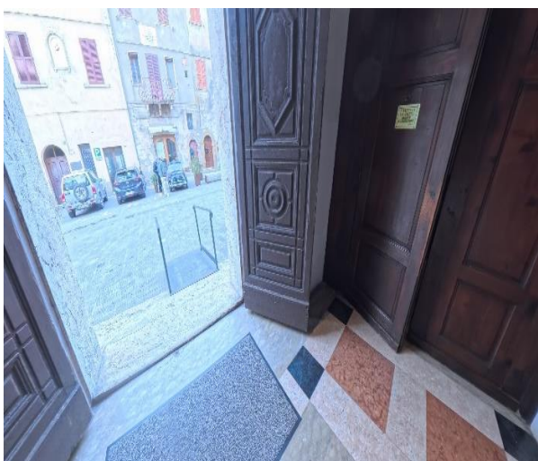
82 interior doors and entrance thresholds
