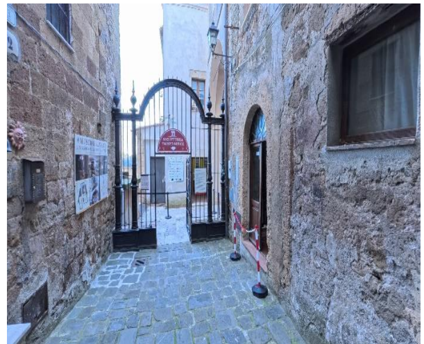
67 Synagogue entrance gate
